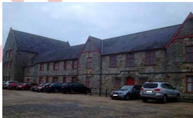
Figure 4.1: Carrickmacross Workhouse, Carrickmacross, Co. Monaghan, Location of the Project's Local Information Centre for Monaghan and Open Day Events Held in Monaghan
